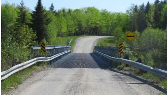
Cardinal Road West Culvert (BCI=71.1 Good)
