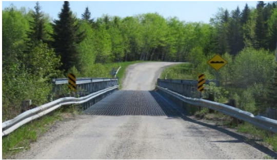
Cardinal Road West Culvert (BCI=71.1 Good)
